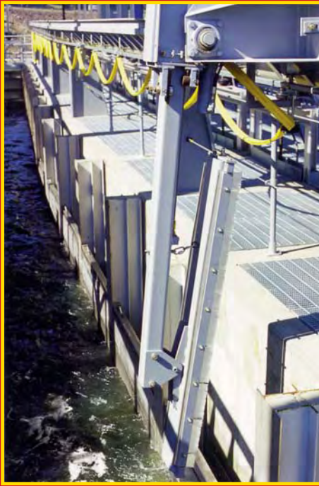
Atlas Polar's new Hydrobrush Cleaning System gently cleans debris from stainless steel intake screens.
