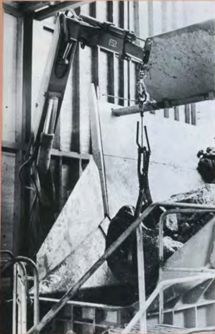
The intake crusher has a HIAB 174 at its side to lift out blocks of stone that are too large or go in broadside on so that the crusher stalls.
