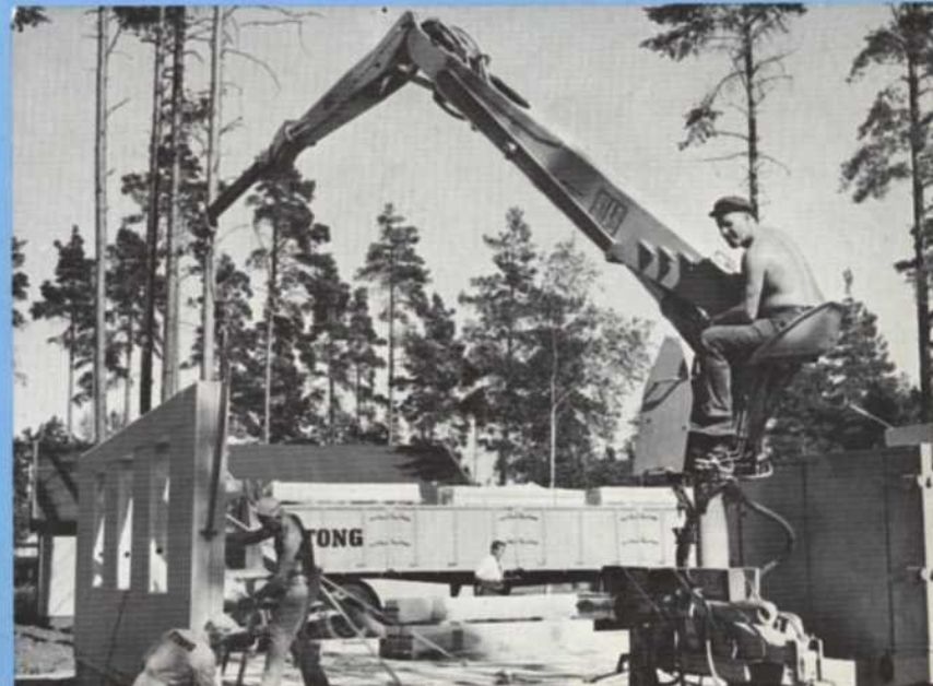
The loader takes the weight of the lintel while it is being positioned above the window opening.
