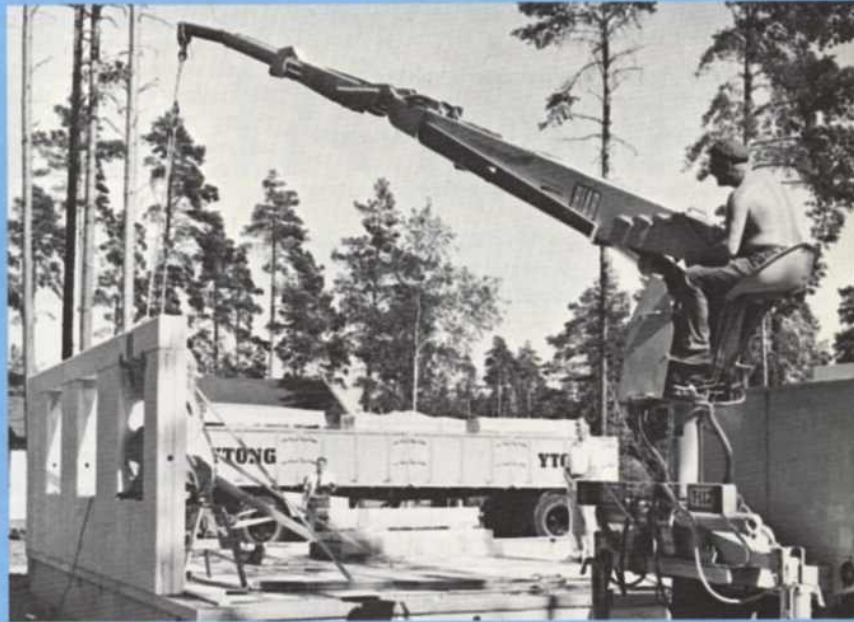
The loader takes the weight of the lintel while it is being positioned above the window opening.
