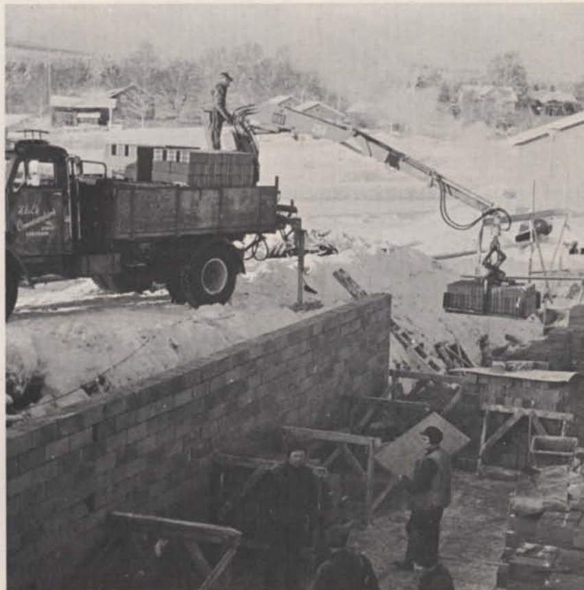
These cement blocks are being handled by a HIAB 174 Speedloader equipped with a special clamp. The driver in the upper picture operates from a control seat sited on the cab roof, giving him an excellent view of the job and making it easier to deposit the pallets just where he wants them. This arrangement also retains the short distance between the front wall of the deck and the back of the cab. The seat is collapsible so as not to make the outfit unnecessarily high. In the lower picture the driver is operating the rear-mounted loader from a special platform. And here we can see just how the blocks are put down right where they are to be used, so that the building workers do not have to bother with unloading at all.
