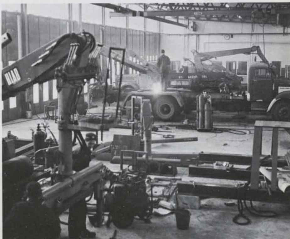
The exuberant growth of HIAB's business in the forestry sector is illustrated by the fact that the Borlänge shop, which was built as late as 1964, was already too small only a year later. The new extension was finished in the autumn of 1966.
