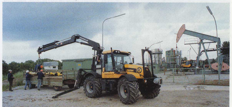
Handling welding apparatus and other equipment in connection with oil exploitation calls for precision. Kremsmüller have what it takes both here and in the construction and servicing of pipelines and pump stations.
