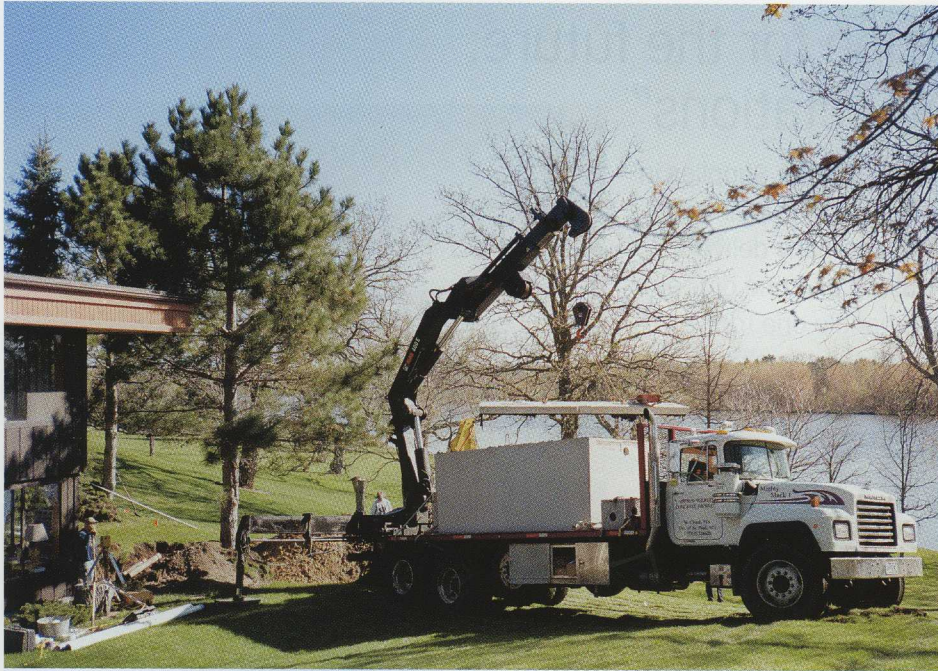
A seven-ton septic tank has to be lifted, from a sloping position, over a pile of earth and then lowered into a pit behind the truck. Tricky? "Well, you run into a lot of this stuff, but with a Hiab 400 it's no problem", says Kevin Ehrlichman.
