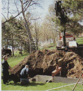
A seven-ton septic tank has to be lifted, from a sloping position, over a pile of earth and then lowered into a pit behind the truck. Tricky? "Well, you run into a lot of this stuff, but with a Hiab 400 it's no problem", says Kevin Ehrlichman.
