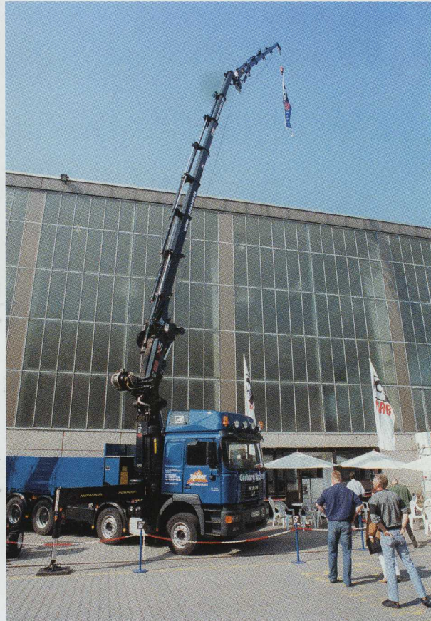
The Hiab flag flew highest at Hamburg's building fair. Delivering roofing materials is a speciality of Gerhard Spöler in Heiden and their new HIAB XS 600 E-7 with Jib-4 reaches nine-storeys high.
