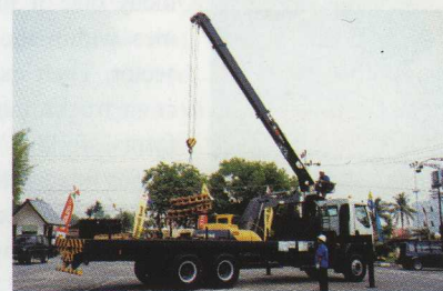
This is one of four HIAB 140 T-4 cranes that PT Siak Zamrud Pusaka use when working on and around Caltex Pacific's oil rigs in Indonesia.
