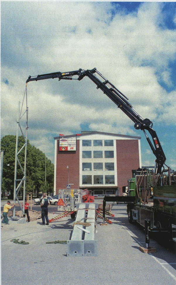
Sven-Olof Jacobsson has been helping to assemble steel constructions for 25 years now. Here, the frame of a lift shaft for a footbridge is being erected.
