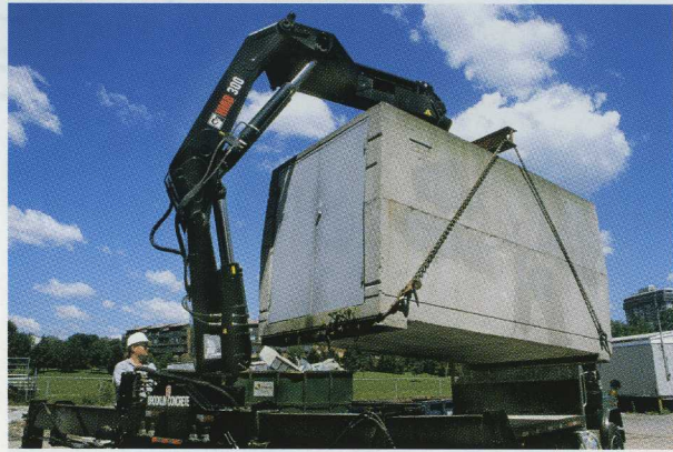
A rear-mounted HIAB 300 affords Brooklin Concrete superb handling in-close during deliveries. And they need the power, because they often handle heavy lifts such as this one – yet another storage vault delivery.
