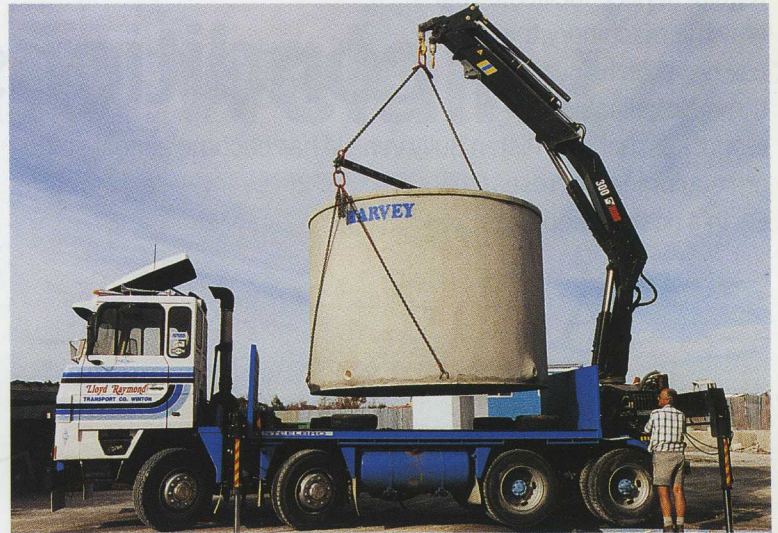
A five cubic metre concrete tank is no match for Lloyd Raymond and his new HIAB 300. He found that placing old tyres as extra shock absorbers under the load made for a smoother ride.
