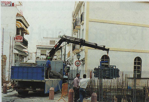
The construction boom is providing everyone with full-time work. Here, Francisco Leyva García of Construcciones Maesle S.L. in Cordoba is making a delivery using the construction firm's own HIAB 095 to an apartment building site in Torremolino.
