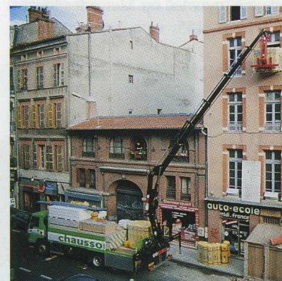
Having put their faith in HIAB cranes, Chausson are pulling well ahead of their competitors in the building materials branch.
