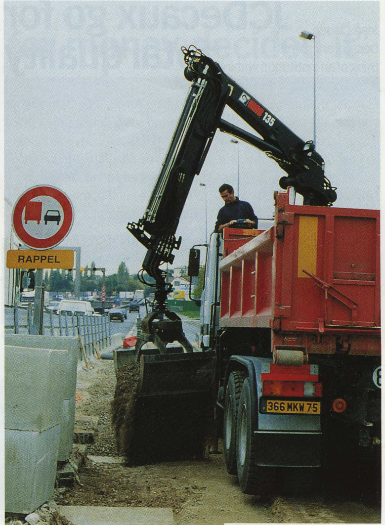
Operator Soares Alvard is laying around the foundations for a noise-protection barrier being erected on the A86 near the Fresne Prison in Paris. He told us he had also used the bucket to load and unload the concrete drums.
