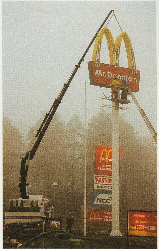
Yet another Golden Arch in position, this time in Hudiksvall. Björn Sjöberg puts them up all over Sweden with his HIAB 195 and its two manual extensions.
