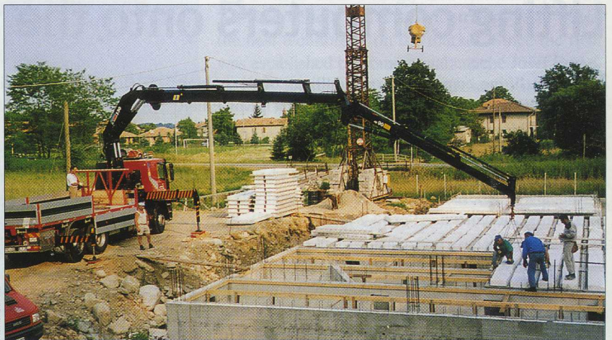
When there's a really difficult job they call for Domenico Curcio. Here he is laying down insulation. The concrete and the frigolit are cast as a single unit, each unit weighing 400 kg. Here one is being placed 16 metres out. The longest reach needed was 22 metres which Domenico managed with the aid of two extra booms and the jib.
