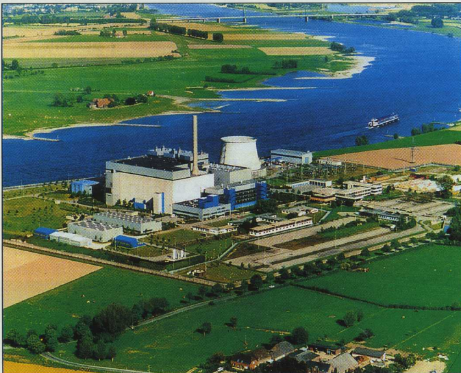
The long disputed Kalkar Nuclear Plant has never been loaded with nuclear fuel. Now it's going to be completely redone with the aid of three new Hiab cranes.
