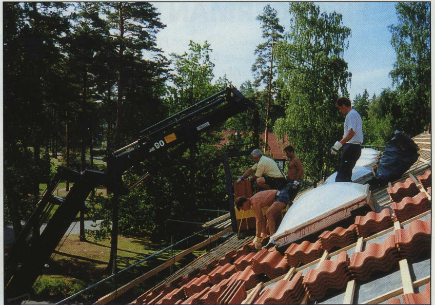
A HIAB 330-5 with jib and rotator made a chore very easy. Lars-Åke Johansson, driver, is standing on the roof, guiding the pallet fork from the truck all the way up to the roof, where the tiles are quickly distributed. Shown is an army barrack in Kristinehamn getting a new roof.
