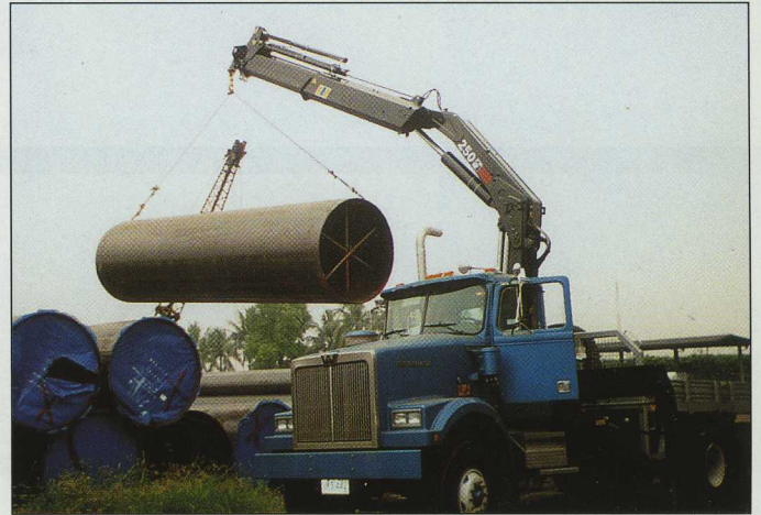
One example of how PNOC uses the HIAB 250-3, here handling large pipe sections.
