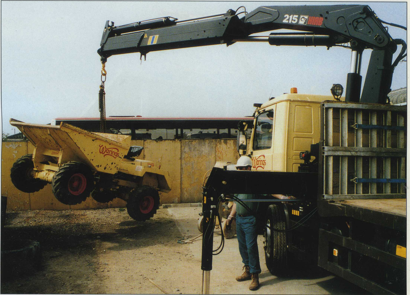
Warings Contractors Ltd countered increasing demands with a HIAB 215-2.
