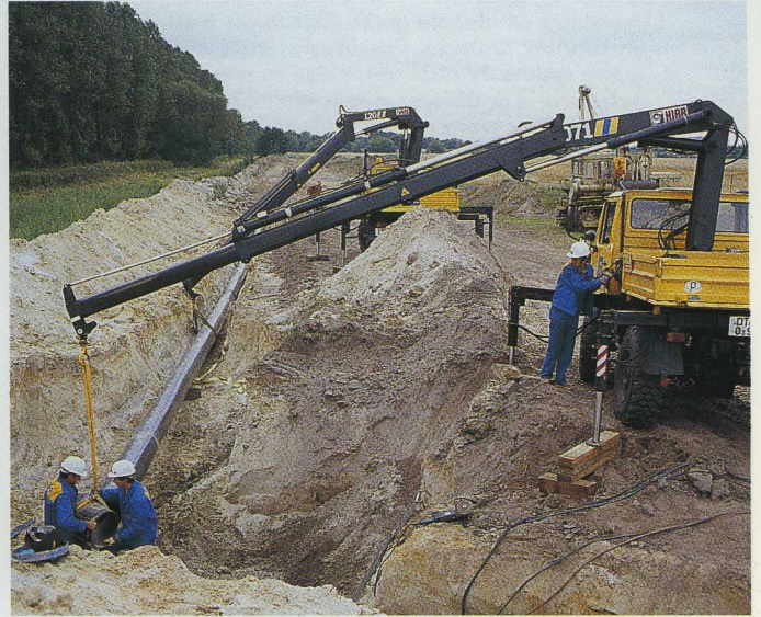
An effective way to lay pipes.
