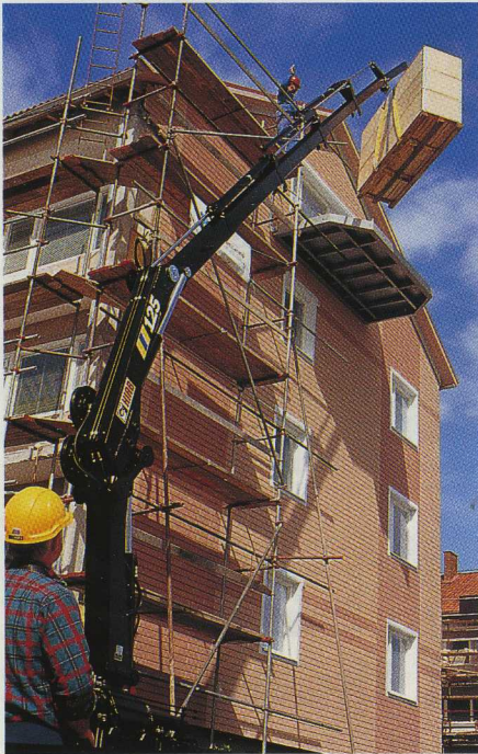
With four hydraulic and one manual extenon, this HIAB 125 has a reach of 14.4 m and is lifting close to 500 kg.
