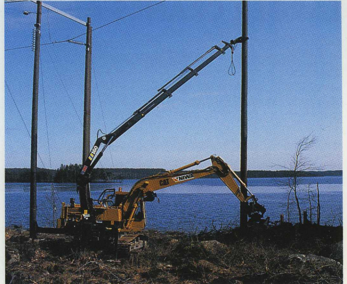
Uddeholm Kraft uses a HIAB 160 mounted on a CAT to maintain their distribution network.
