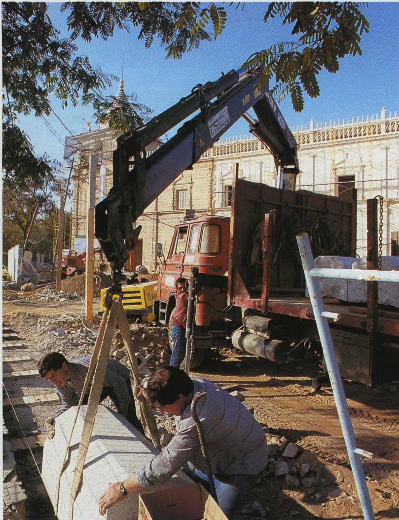
There's also a lot of construction going on outside the EXPO '92 grounds. This HIAB 140 AW mounted on a Spanish built Barreiros truck, owned by Isidoro Gonzalez & Sons, is being used to unload and position heavy granite stones that will form part of a fence around the new Andalusian Parliament buildings in Seville.
