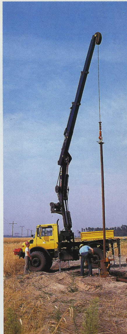
Polluted water must be pumped out of the ground.
