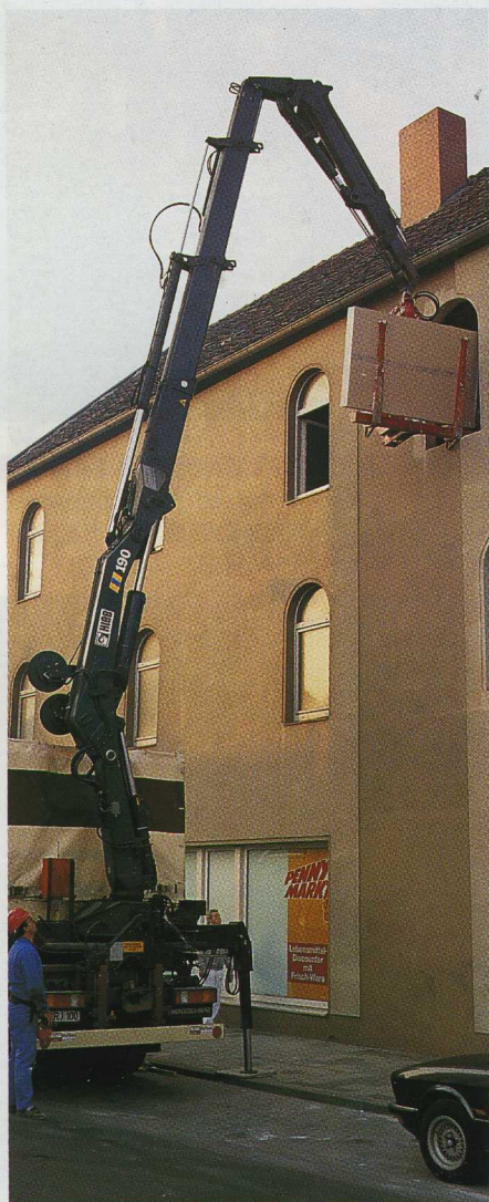
Cargo is easily deposited on the third, or fourth floor.
