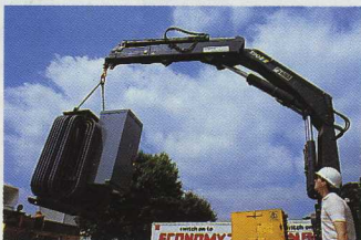
Transformers are loaded and unloaded with HIAB 260 AWWs.
