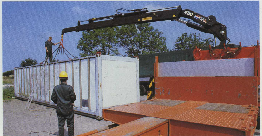
THE HIAB 450: An effective and less expensive alternative to mobile cranes
