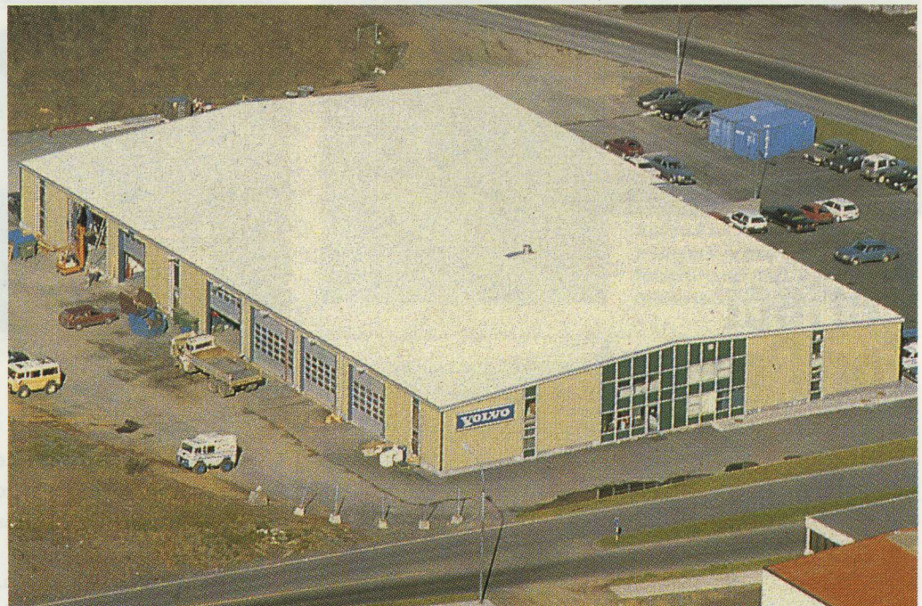
Brimborg's service center in Reykjavik.
