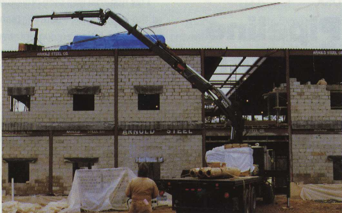
HIAB's DigiDrive offers the operator full mobility for an unobstructed view of his lifting operation.
