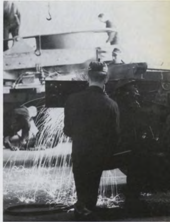
Major modifications often have to be carried out on chassis. This frame is being cut short so that it can be fitted with an auxiliary frame before the tipper deck is mounted.
