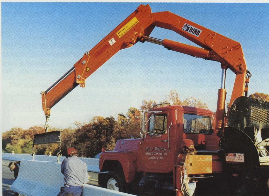
The flexible action pattern of the HIAB crane permits the fast and exact positioning of the units.
