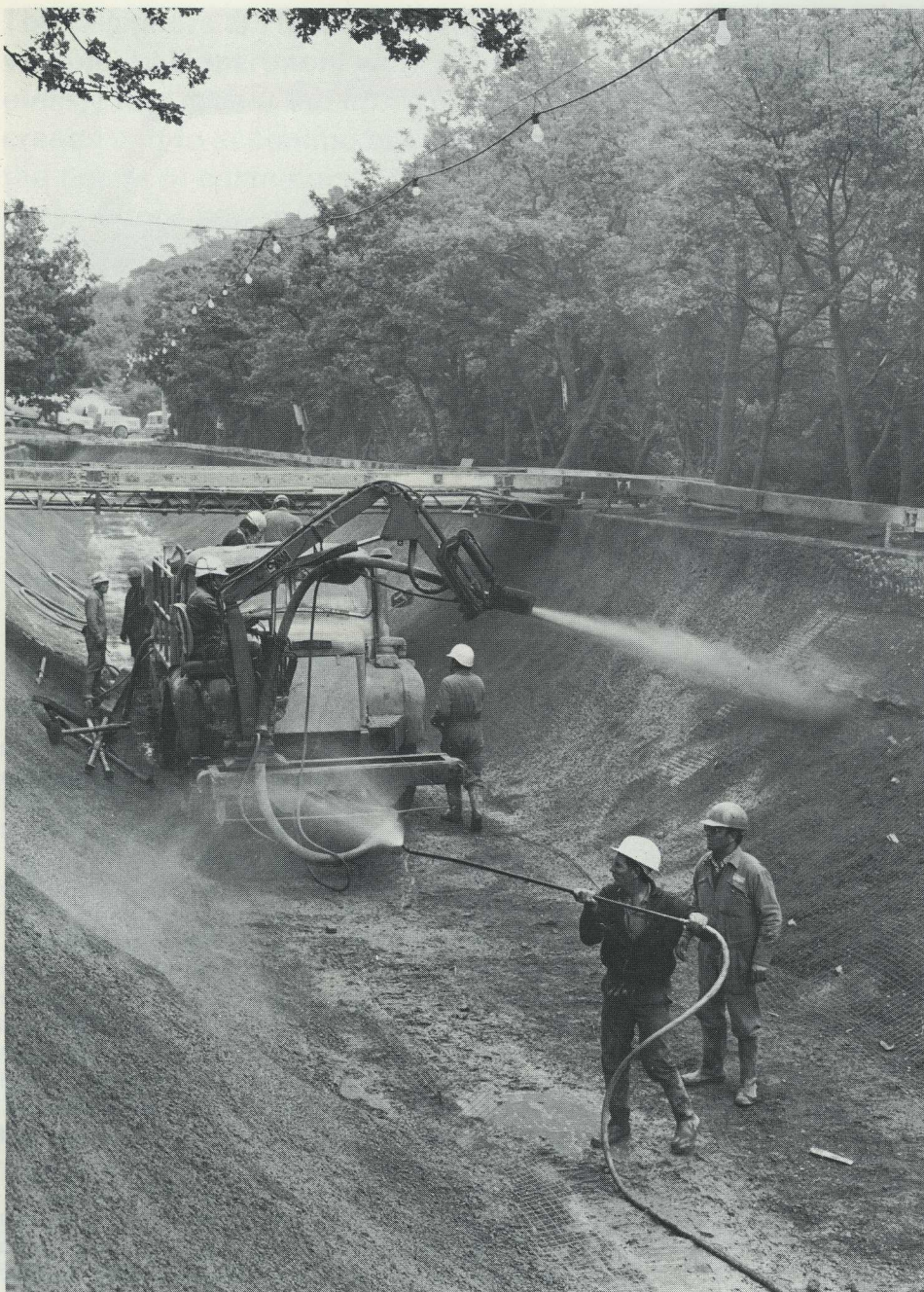
The concrete for the gunite units is transported on the monorail track visible in the background and is filled from the bin rear-mounted on the guniting vehicle.
