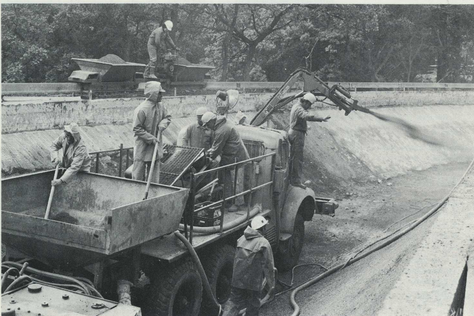
The concrete for the gunite units is transported on the monorail track visible in the background and is filled from the bin rear-mounted on the guniting vehicle.
