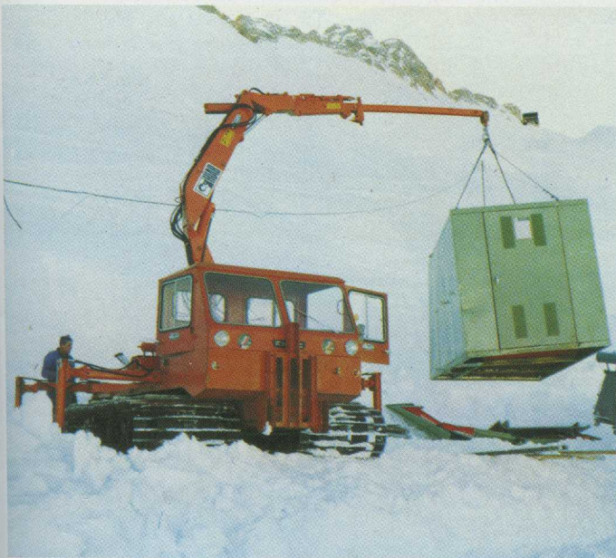
And here they've just set up a hut for the cableway crew. Again: the HIAB loader did the lifting.
