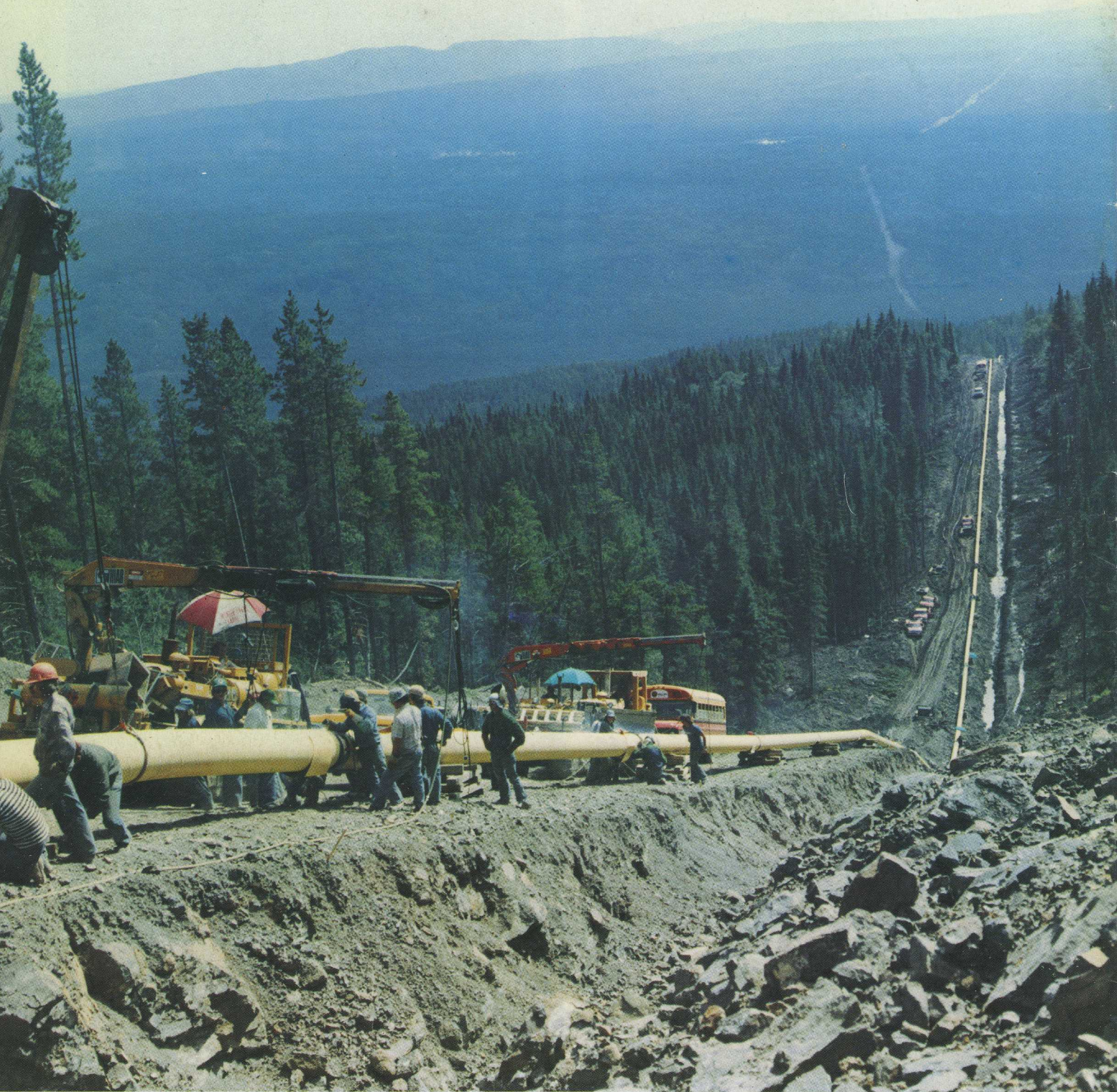
This awesome view is from Grizzly Valley in north-eastern Canada, where the HIAB Method is being used on a big pipeline contract in very difficult terrain far out in the wilds. More about it on page 7.
