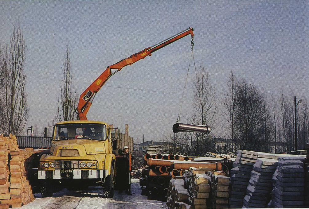
The state enterprise ELBUD builds the high-tension lines that criss-cross Poland. It does much of its materials handling by the HIAB Method. These pictures show the loading of pipes onto a Fiat/Unic by a HIAB 550 (above) and of transformers (below).
