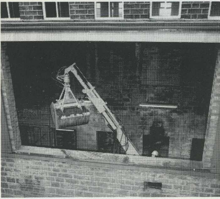
Through an opening in the exterior wall the slurry can be passed straight out to a waiting lorry.
