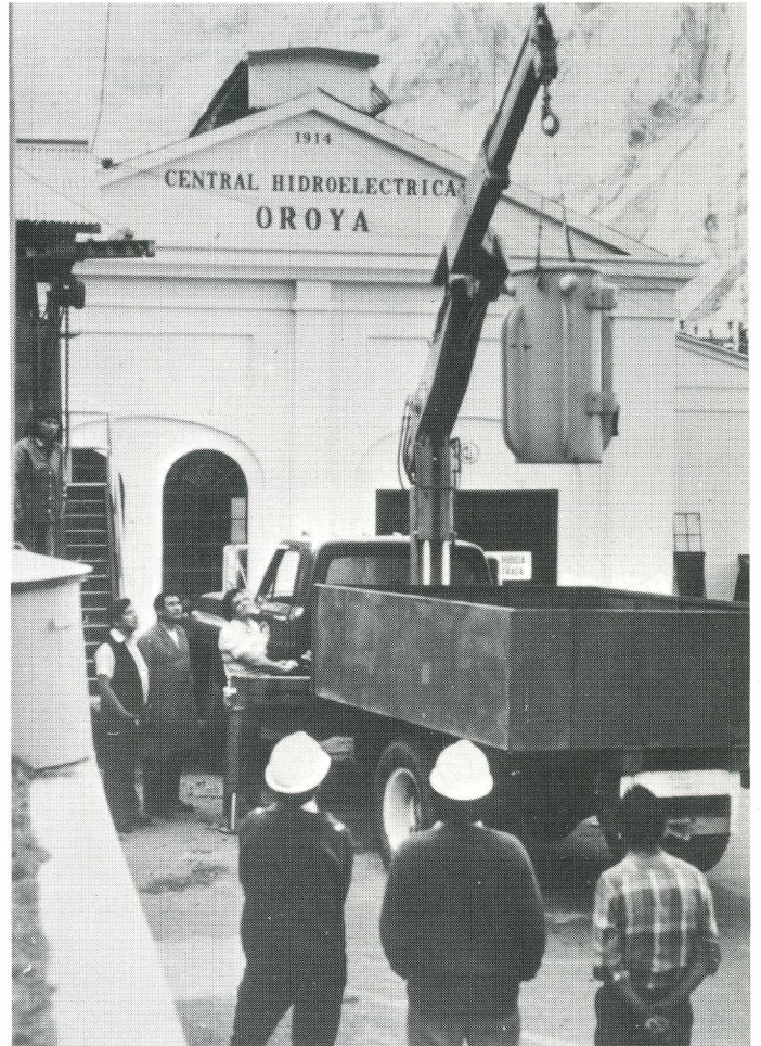
All the heavy equipment at an oil refinery in Bayovar, like this 2.5-ton diesel set, is handled by a HIAB 950 (above). On the right, a HIAB 950 hoists a transformer in Oroya. A HIAB 550 with a personnel basket (below) is used by the electricity works in Chiclayo for such tasks as cleaning insulators.
