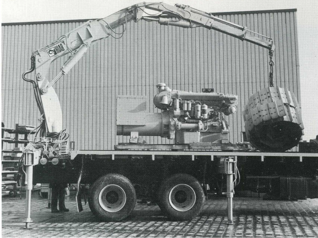
An extra pair of outrigger legs provide stability for the heavy lifts.
