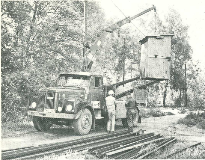
The first job of the day is to collect the welding equipment, which is kept in a hut. Åke hoists it onto his truck — hut and all.
