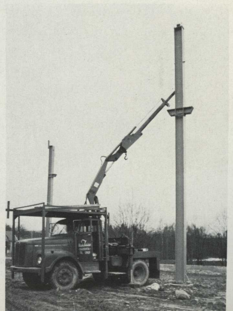
Many buildings are erected throughout by HIAB loaders, from the first post in the framing to the last wall sheet.
