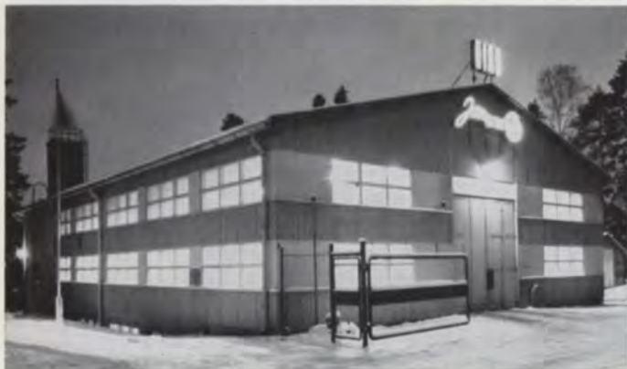
The new repair and service shop in Sockenbacka has a floor-space of 4,300 sq.ft.
