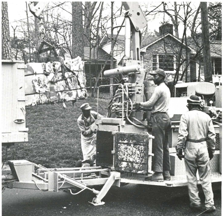
Collection is usually the most costly stage in dealing with refuse. Winston Salem has tackled the rising costs by mechanisation. The refuse bins are collected by a rubber-tired cart, and both the cart and the bin are lifted hydraulically for emptying.
