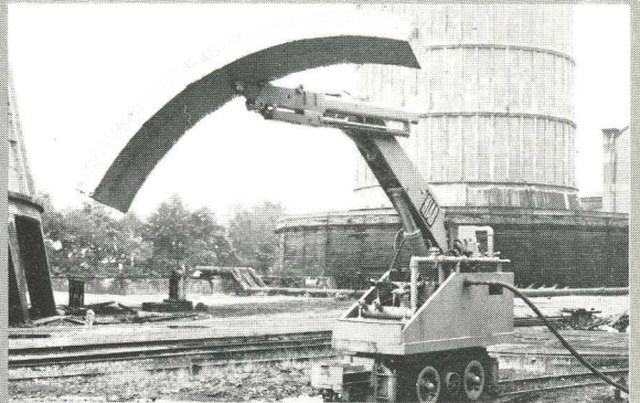
3 The swivel bolt by which the concrete unit is hoisted is located at the C.G. so that the unit balances in all planes.
