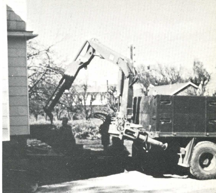
The heaviest stairways which Lennart Arvidsson handles weigh three tons, but the Hiab 950 can take the weight and outrigger legs give it the stability needed for spotting the stairway exactly in position.
