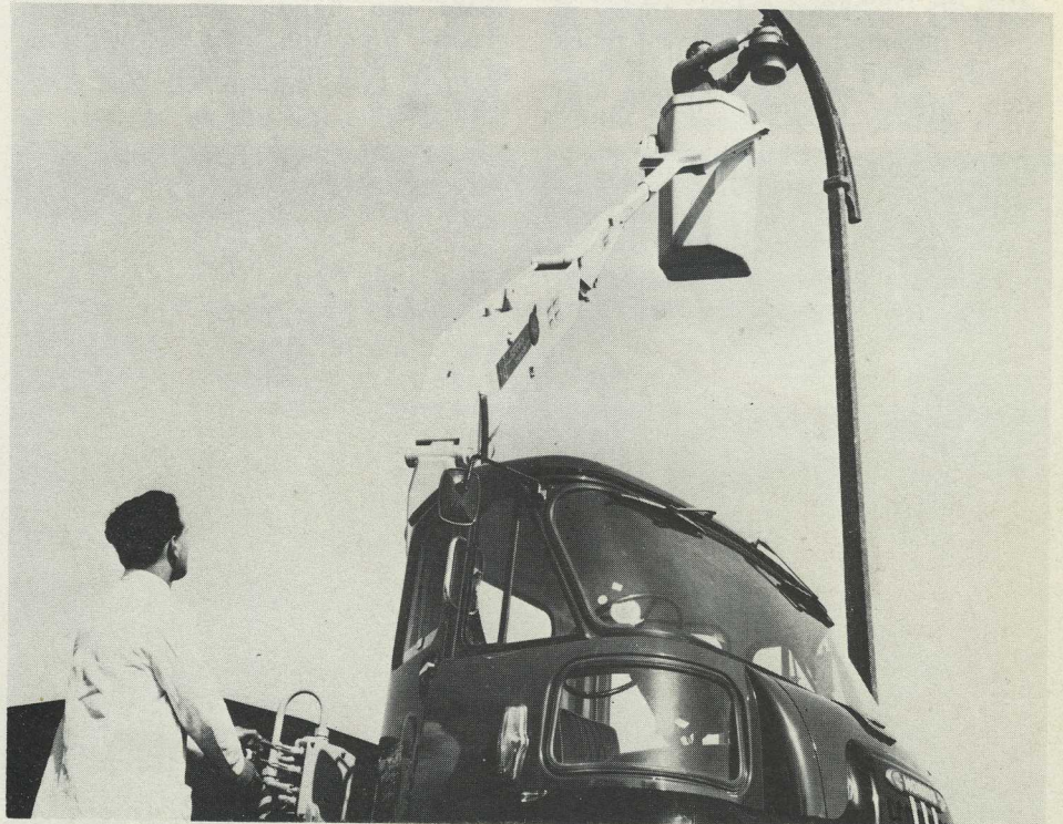
A Hiab loader with a personnel basket is a very common and very serviceable piece of equipment, saving a great deal of time in maintenance work on street lighting and overhead power lines.
