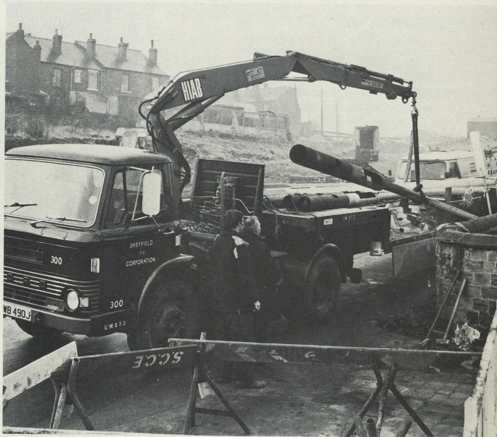
In this way, four men can raise 8—10 standards a day. The old method required an eight-man crew, who could only manage 2—3 standards a day.
