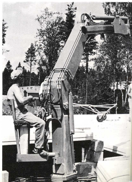
The HIAB 2451 is used for both loading and unloading concrete beams at the precast-concrete works in Östra Grevie.
