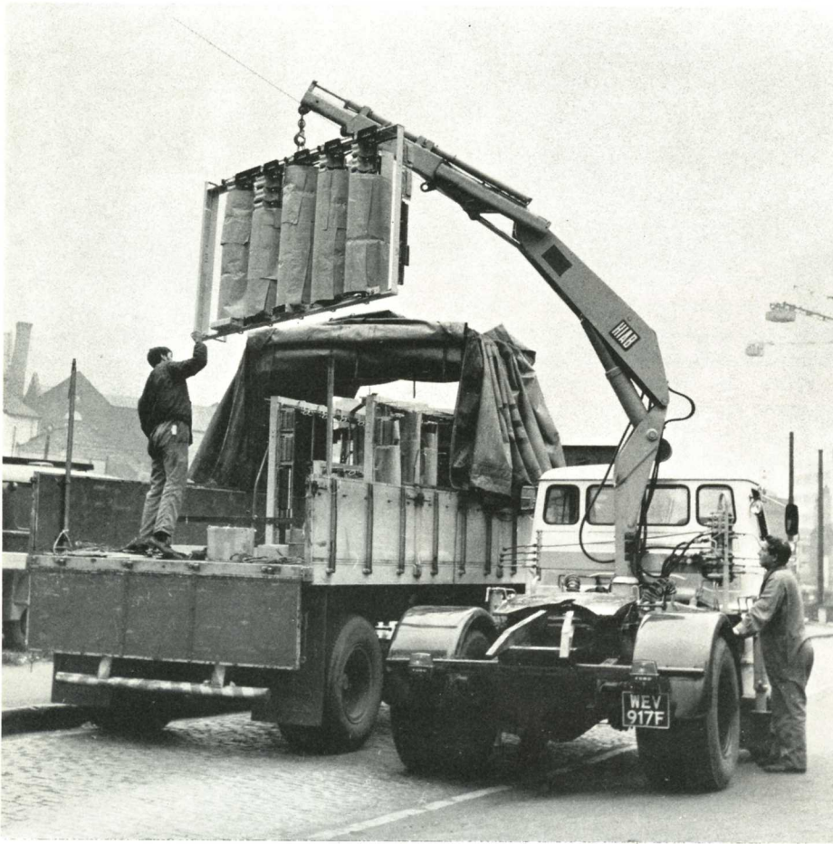
Unloading and transporting a rack to the site of a telephone exchange takes only about nine minutes with the Hiab Method and two men as compared with 45 minutes and 6-10 men with the method previously used.
