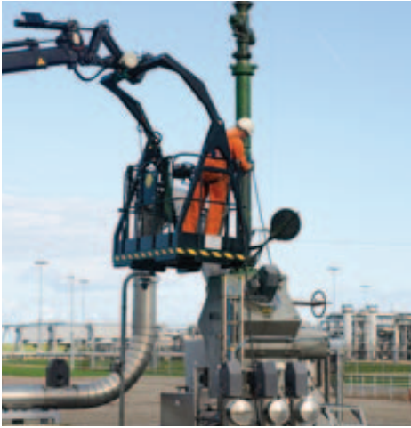
The remote radio control system is ATEX certified and enables the operator in the MEWP to control the crane and installation process on top of the Xmas tree with extreme precision.
